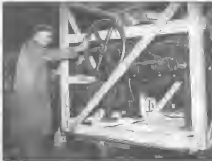
FIRST REPARATIONS FOR BRITAIN FROM GERMANY were landed at Tilbury Docks, Essex, in December 1946, consisting of secret drawing presses which enabled the Germans to substitute steel for brass in the manufacture of heavy cartridge cases. The machinery came from a Hamburg factory that escaped damage from the R.A.F.'s attacks during the war.
